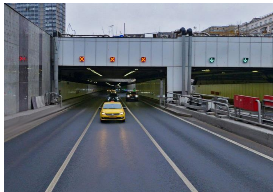
Volokalamsky tunnel (Moscow, RF)
