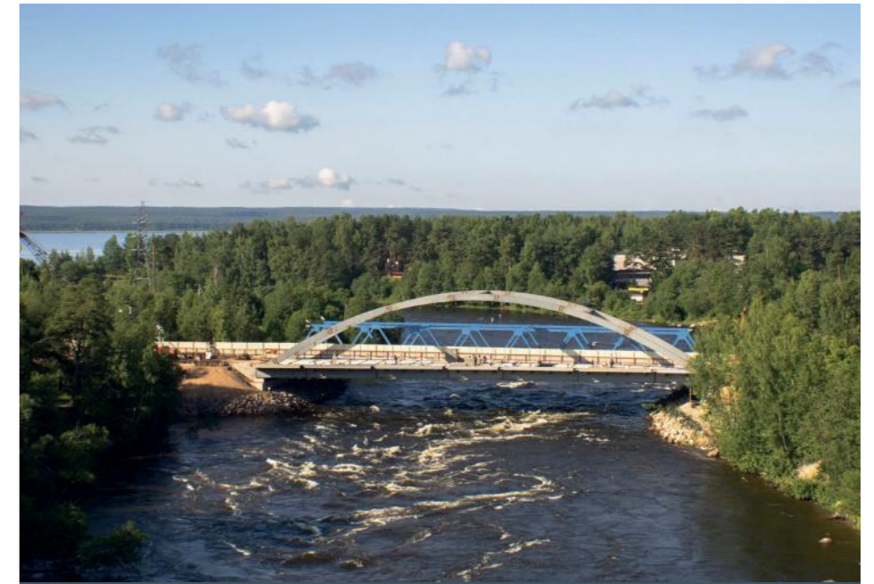
Bridge across the Vuoksa River (Leningrad Region, RF)
