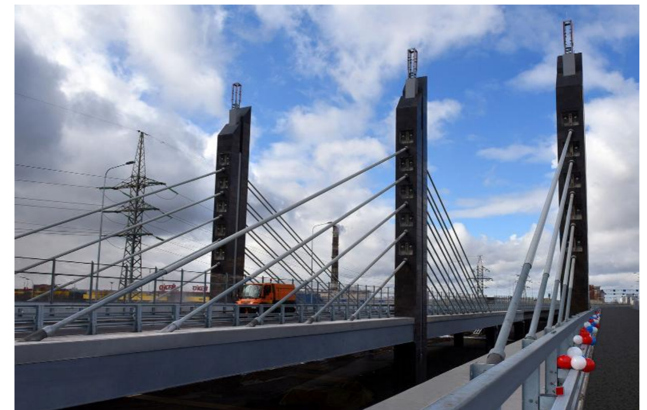
The overpass on Dunaysky Prospekt (St. Petersburg, RF)
