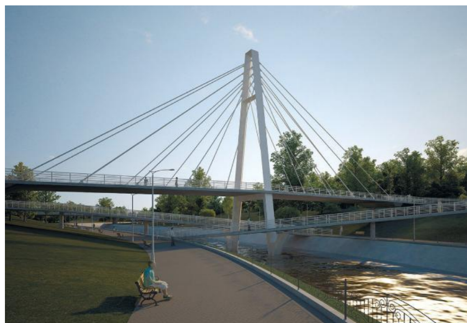
Cable-stayed footbridge (Tashkent, Uzbekistan)
