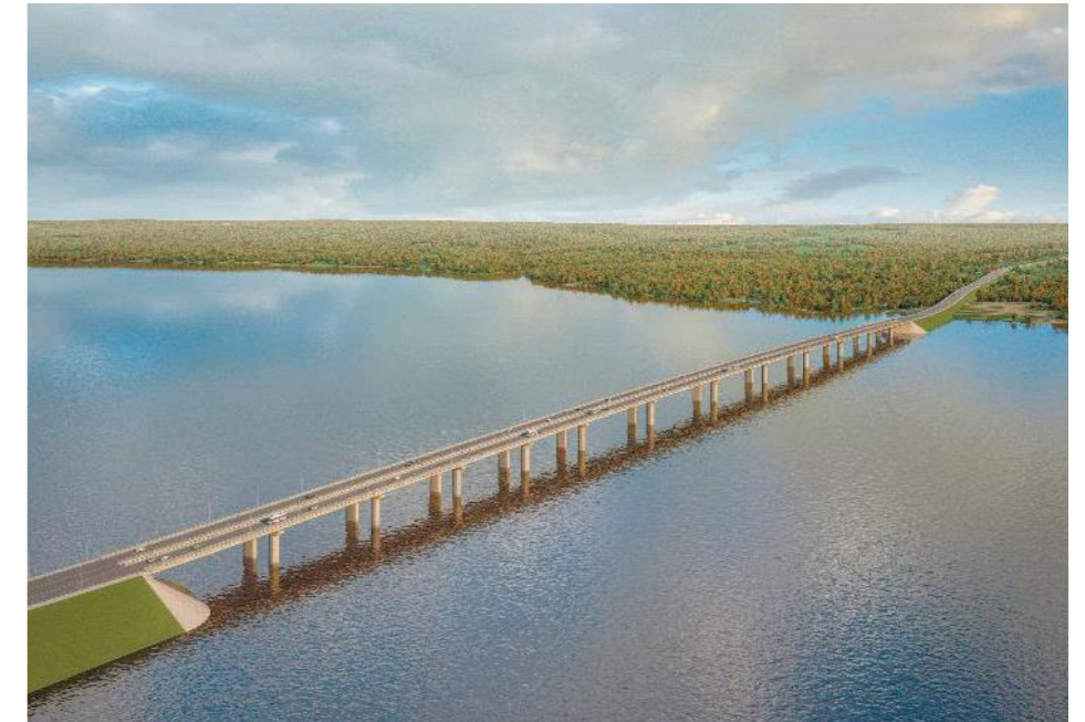
Bridge crossing over the Chusovaya River (Perm, RF)
