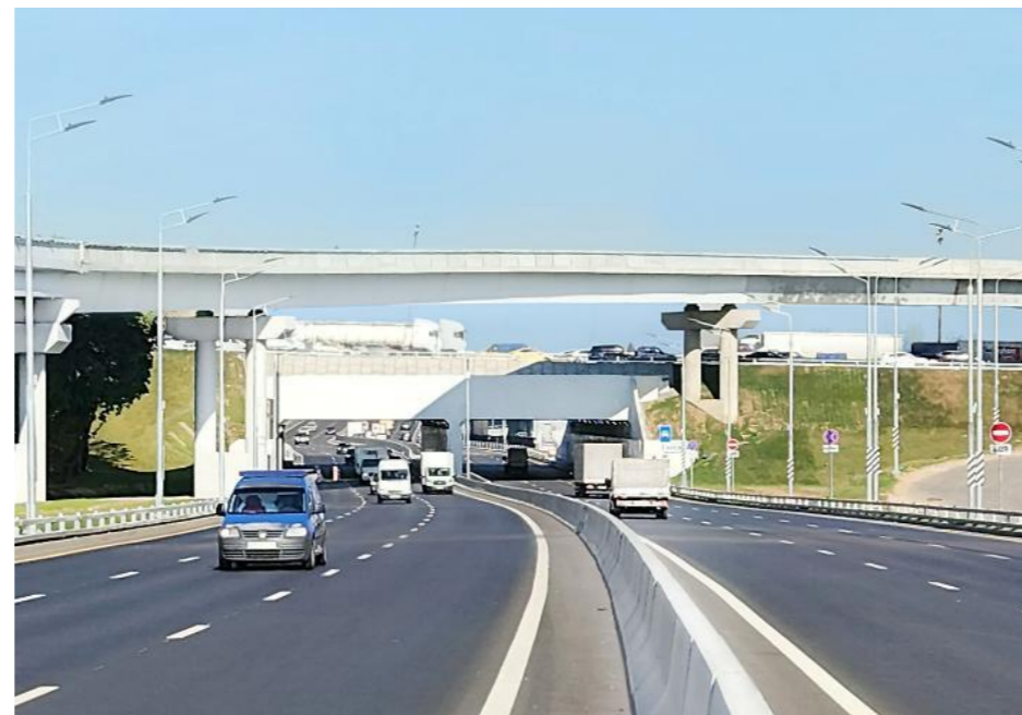
Tunnel Moscow high-speed diameter (Moscow, RF)
