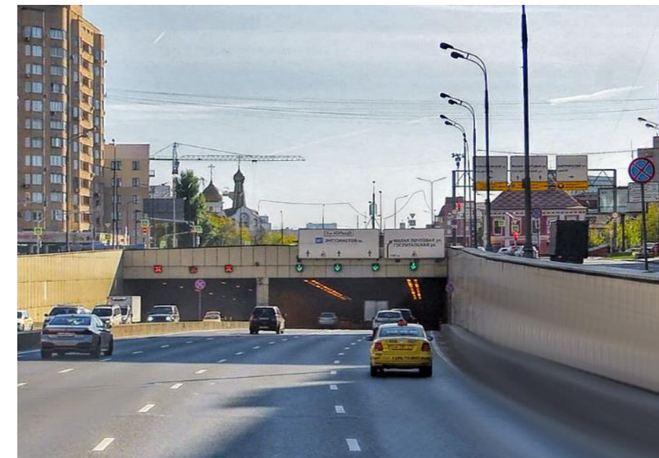
Lefortovskiy tunnel (Moscow, RF)
