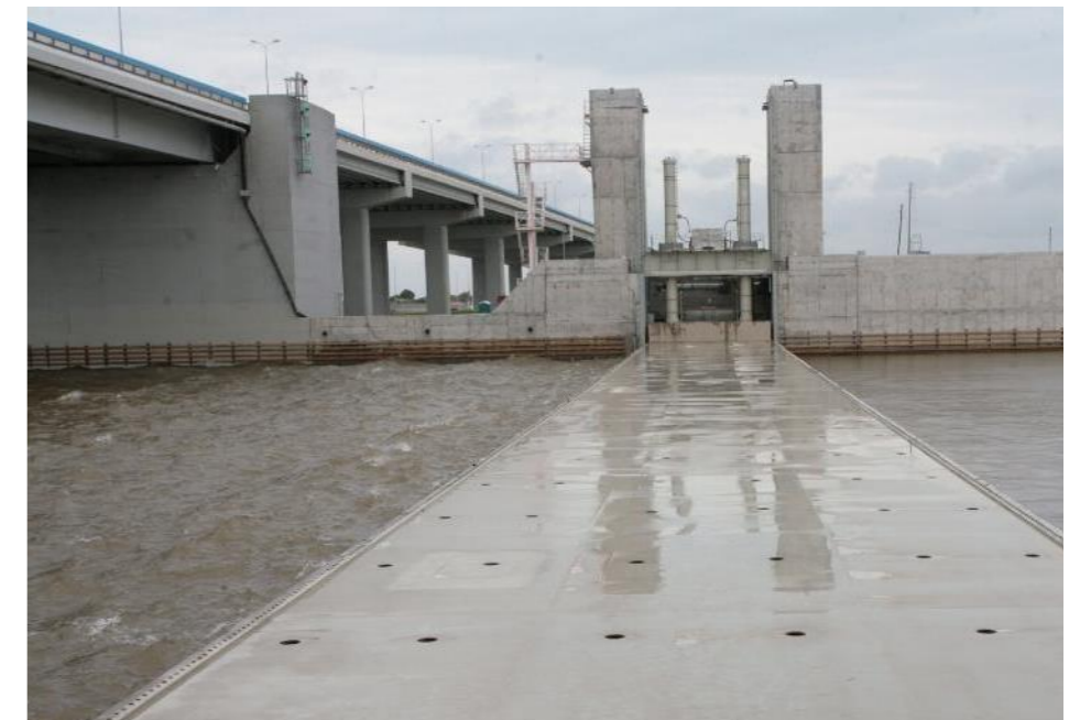
Navigation pass C-2 in complex of flood protective structures (St. Petersburg RF)
