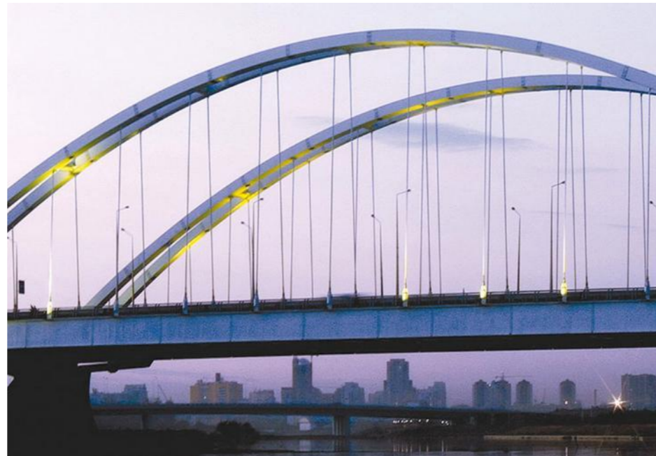
Bridge across the Ishim River (Astana, Kazakhstan)
