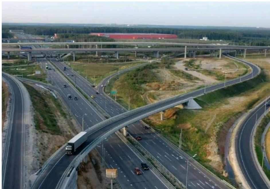
Central Ring Road, the Moscow Region, 1 st stage, section 1 (Moscow, RF)
