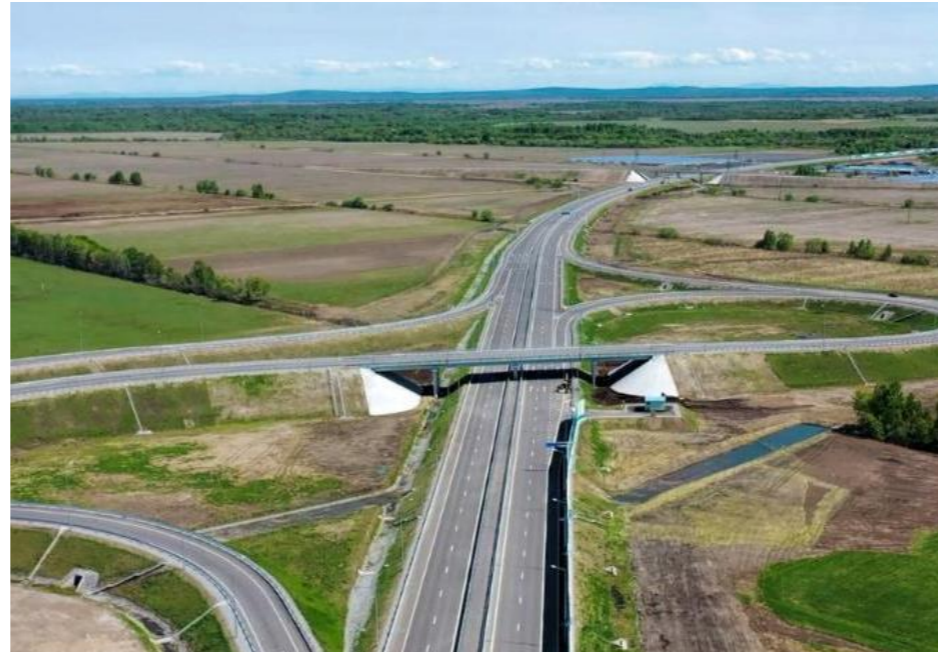
Ring Road over Khabarovsk City on 13-42 km (RF)
