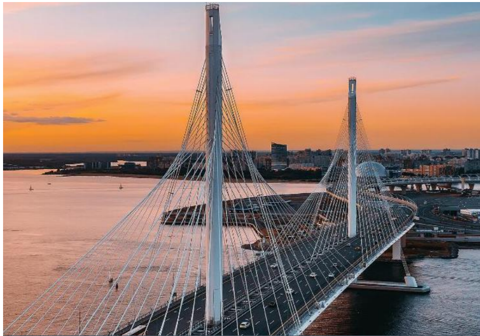
Bridge across the Petrovsky Channe (St. Petersburg, RF)
