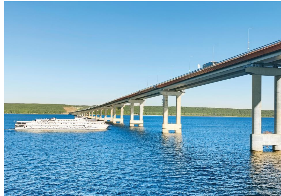
Bridge over the Volga River (Tatarstan, RF)
