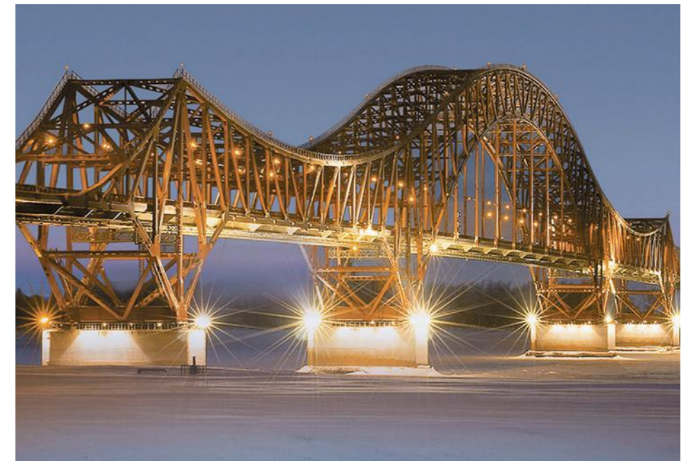
Bridge across the Irtysh River (Khanty-Mansiysk, RF)
