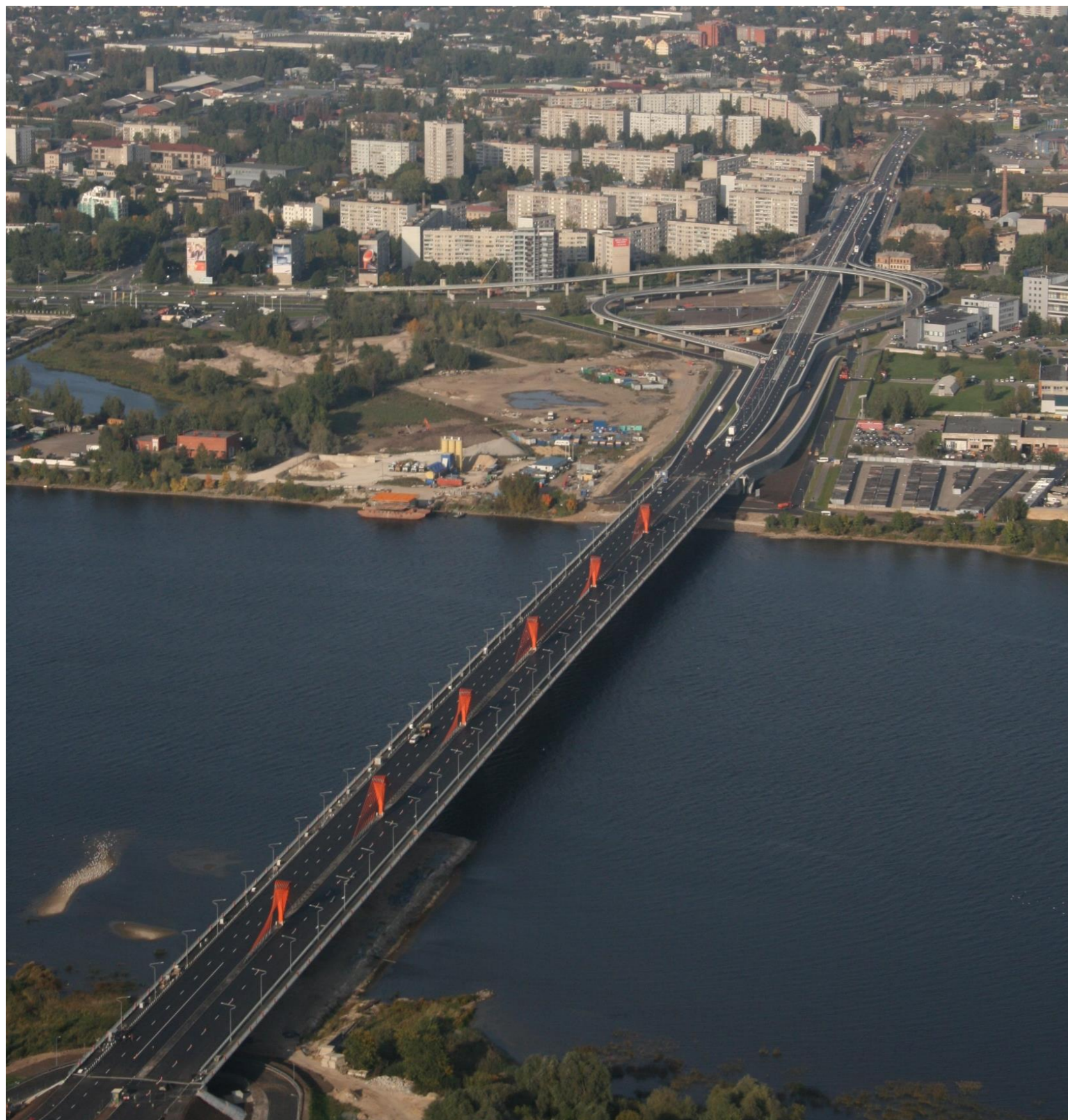
South Bridge over the Daugava River (Riga, Latvia)
