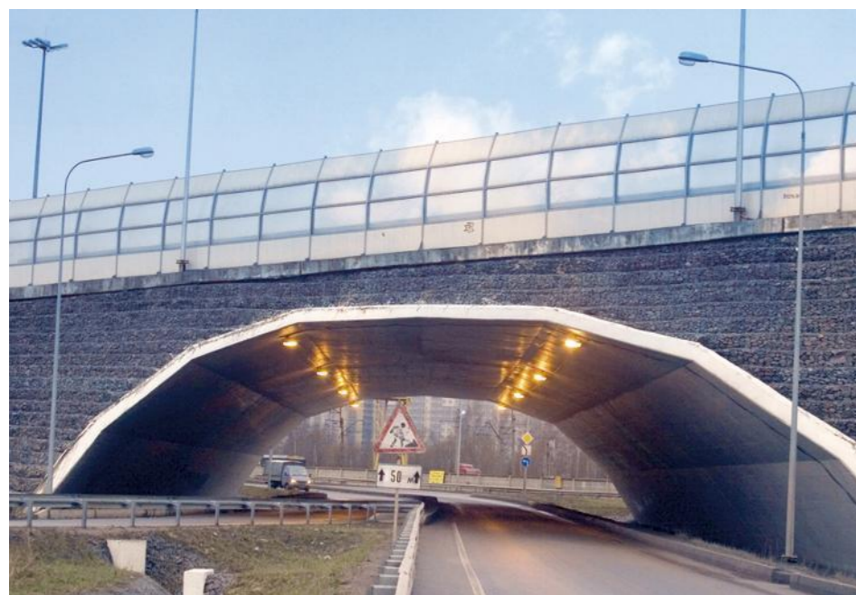
Murinskiy tunnel (St. Petersburg, RF)
