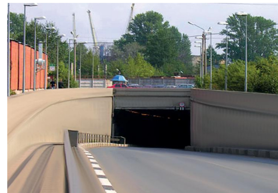
Kanonersky tunnel (St. Petersburg, RF)
