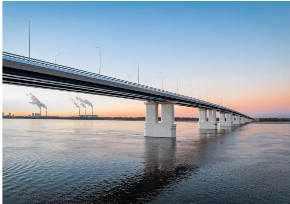
Bridge crossing over the Ob River (Surgut)
