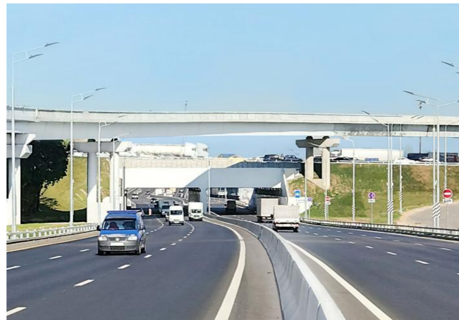
Tunnel Moscow high-speed diameter (Moscow, RF)
