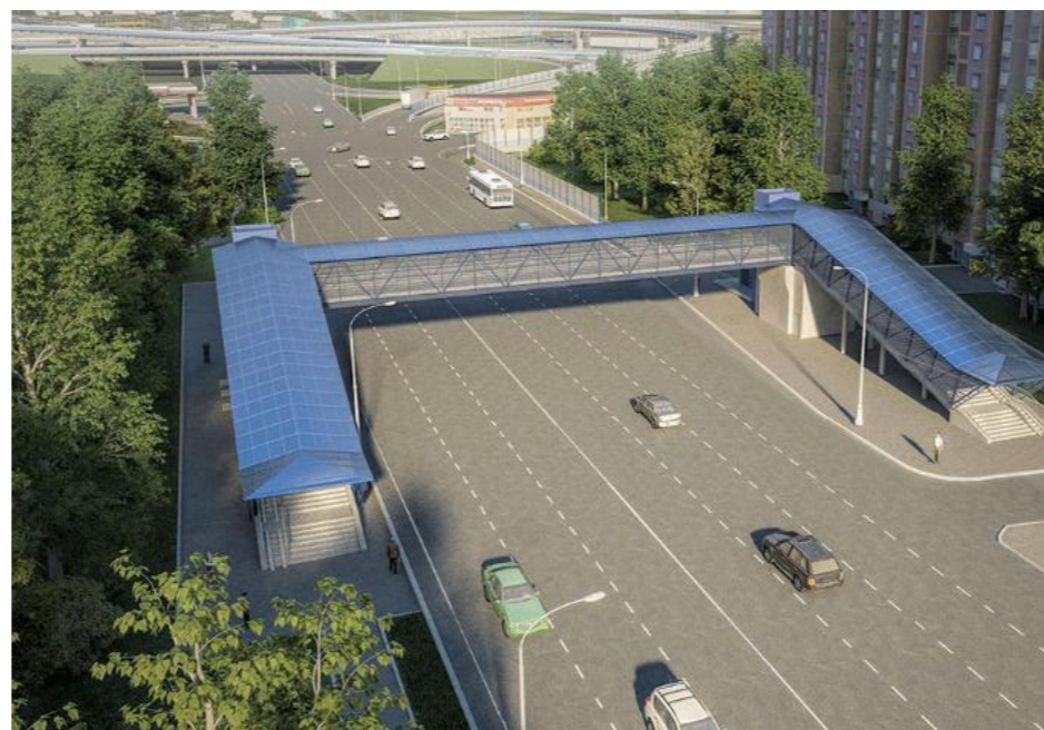
Archway pedestrian crossing (Moscow, RF)
