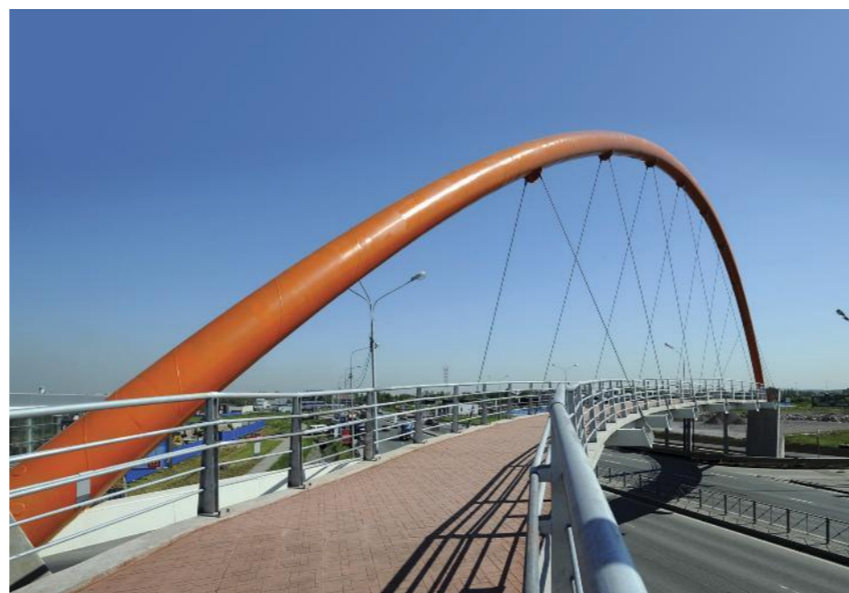
Footbridge on Tallinskoe highway (St. Petersburg, RF)
