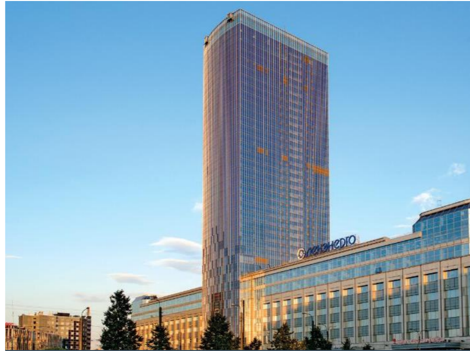
Multifunctional data Center on Leninsky Avenue (St. Petersburg, RF)
