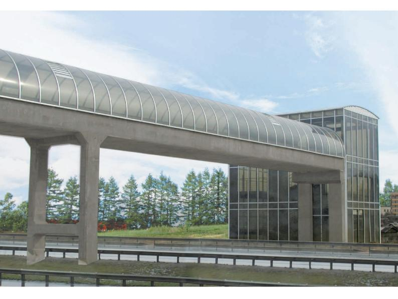
This structure was design as a pedestrian crossing prestressed deck with intermediate pier connected to deck via truss girder. Temperature gradient was considered within abutments located on the ground areas. Pedestrian viaduct was completed by concreting procedures on service bridge as a solid prestressed RC structure with protective layer of polycarbonate.
